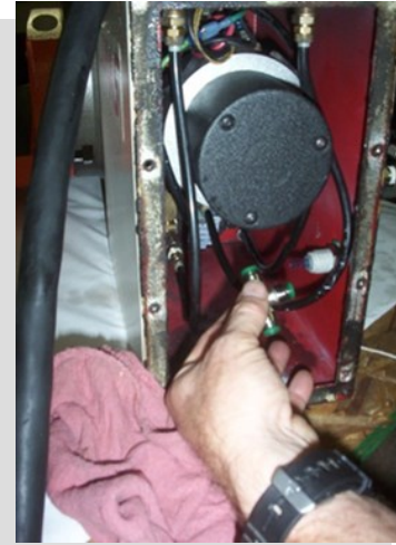
3. Cut this hose in half as close to the opening of the box as possible and attach quick disconnect "T" (provided)
